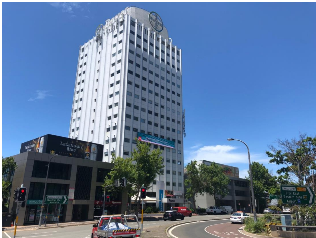
Figure 5 – Built form along Alfred Street
