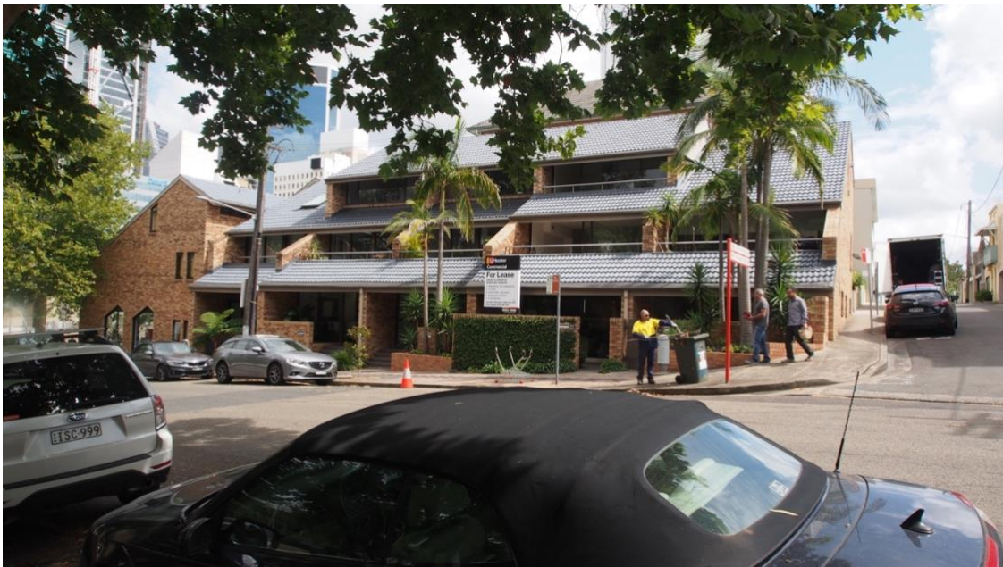
Figure 6 – Southern boundary of precinct Source: Grimshaw
